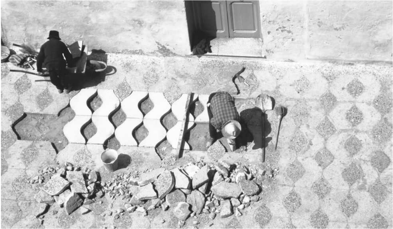
Workers replacing tiles on a Moroccan street.
